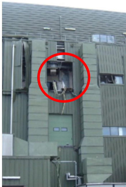
Figure 1: The north side of production Building No. 2 (PB2), post-incident, with the upper roller-shutter door missing (circled). Image source: Loss Prevention Bulletin
